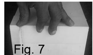
Repeat this process on the other three corners. When installing the frame, care should be taken not to allow mechanical corners to come apart.
