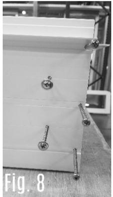
After the jambs are adhered to the sill and head use the packaged screws to insert into the predrilled holes in the jambs and fasten (Fig 8). Use the 8 x 2 ½ pan head screws in the outer holes and the 8 x 2 ½ round washer head screws in the inner holes, do not over tork.
