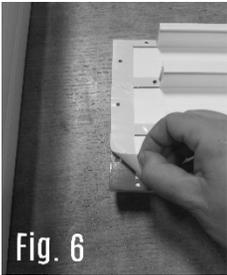
Be sure to assemble the frame one corner at a time. Saw horses are recommended to keep the frame profiles off the ground and safe from damage during assembly. You will notice that the butt ends of the frame have joining gaskets, using the provided alcohol wipes (Fig 5), clean the area where the jambs gaskets will be adhering to the head and sill. Remove the liner from the gasket (Fig 6), align the jamb to the sill and press together (Fig 7). Repeat the steps for the jamb to header.
